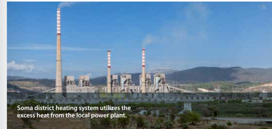
Close cooperation between the Technical Department of the Soma Municipality and Danfoss to make the district heating system a success.
